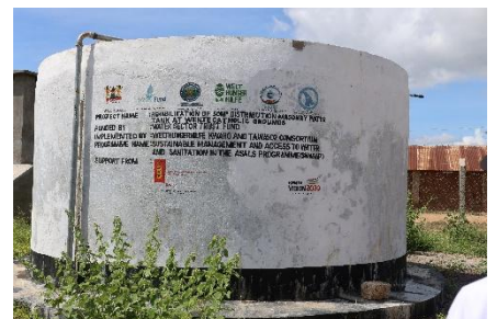
Rehabilitated 50m³ Masonry tank under Wenje-Vukoni Water Project
